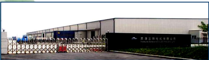
Tianjin Samwha Electric #1 plant (China) – Green Cap (EDLC), E-cap (Snap-in,Screw,Radial)
